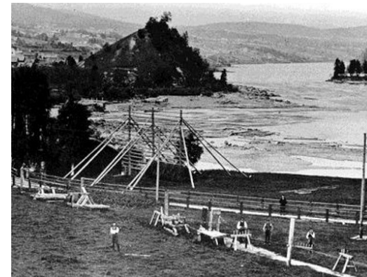
Big structure for drying hay
