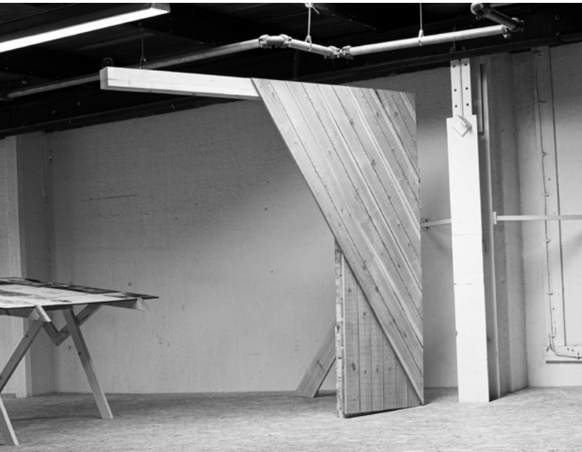
Detail of loadbearing columns made of CLT with diagonal board to ensure rigidity / Photo of 1:1
