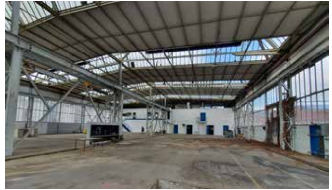
KHD inspection hall inside
