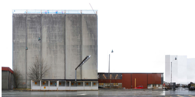
Street elevation of the BAS site and building
