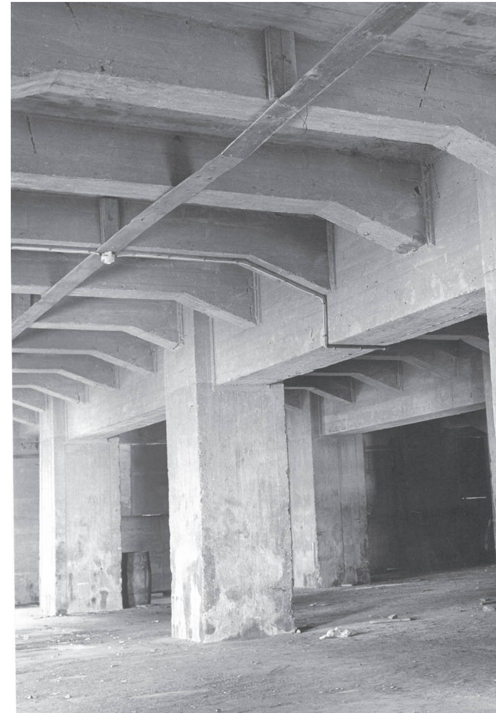
Reinforced concrete columns 1x1meter groundfloor
