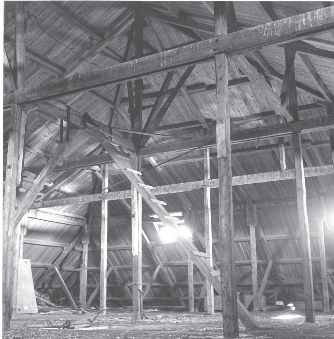
Wood construction on the loft
