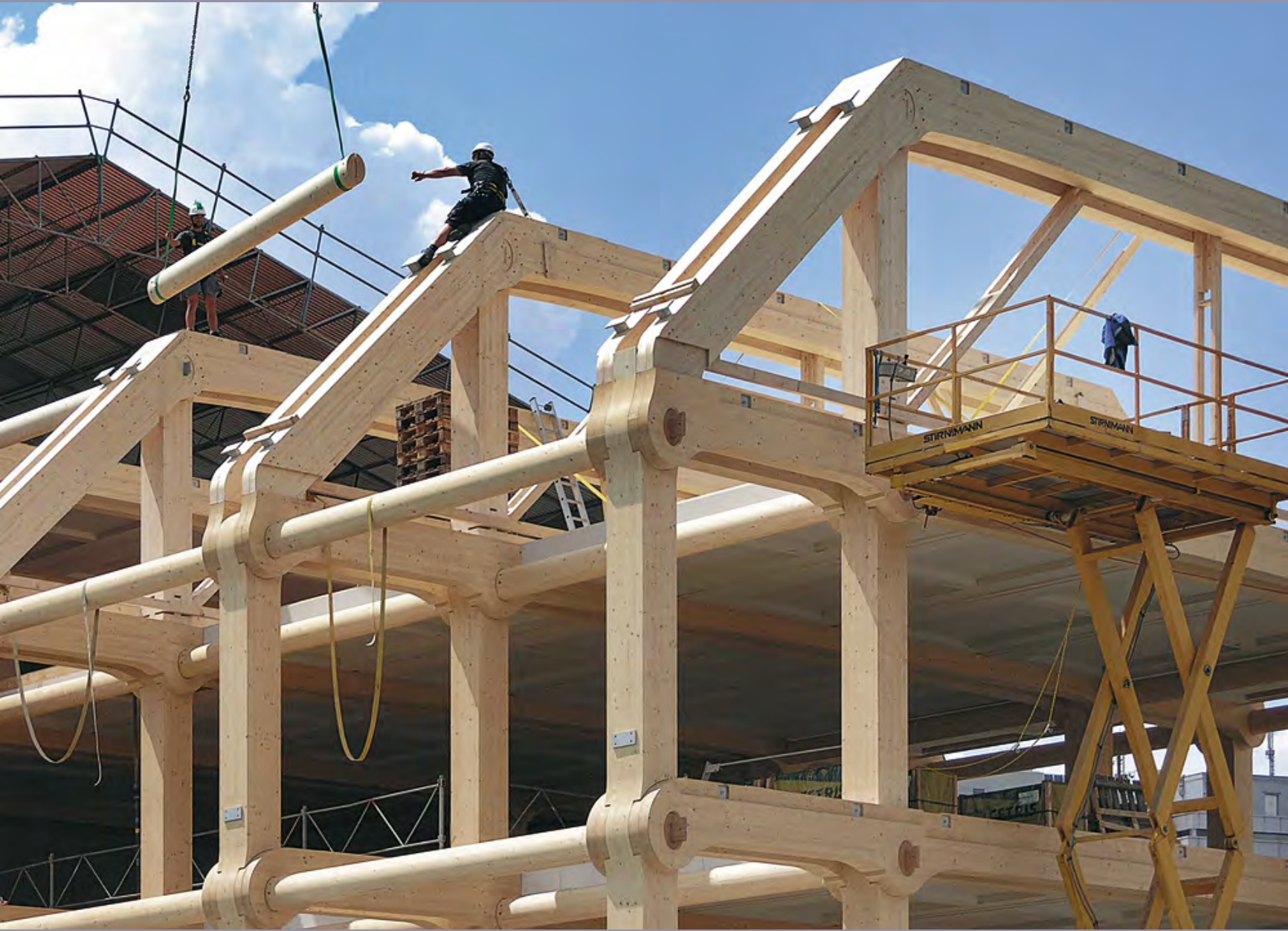
Show Off! Large scale wood-joinery. Media house Tamedia publishing house in Zurich, architect Shigeru Ban
