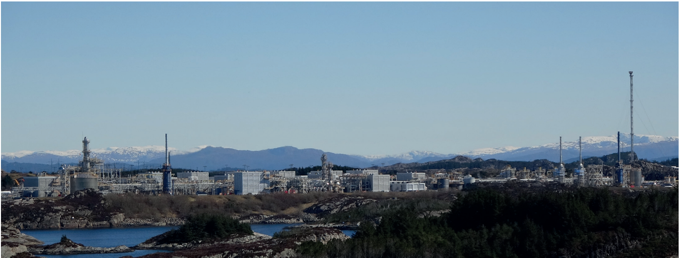
Kollsnes, a gaz processing plant. Personal photography
