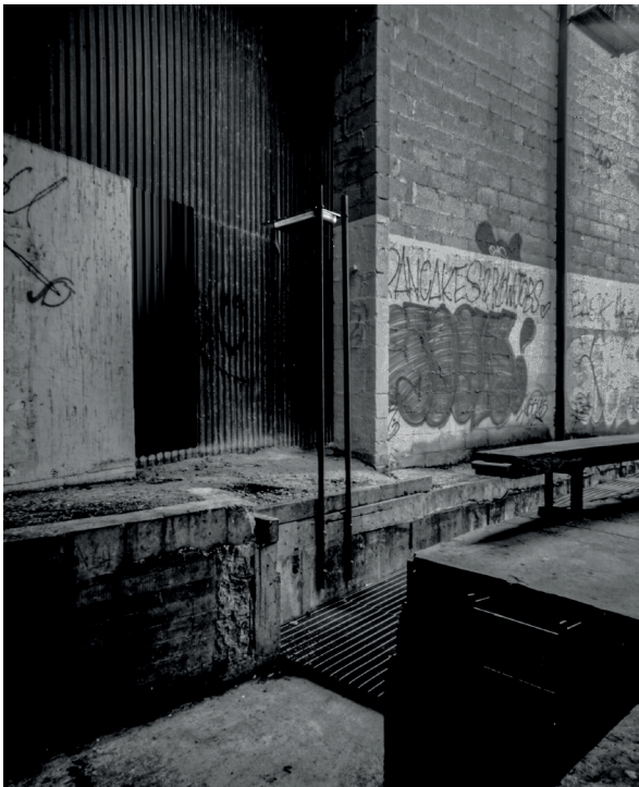
Behind the water container is the firewall and the neighbour's wall. Left are the basement doors and right is the waterfront. Top right is the emergency staircase and in our backs is the dead-end. The nests are above.
