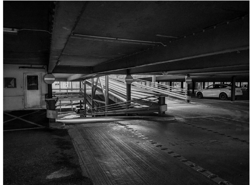
Circulation ramp for cars
