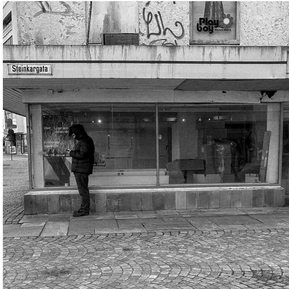
The presence of vacant shop windows contributes to the perception of the site as lifeless and inactive.
