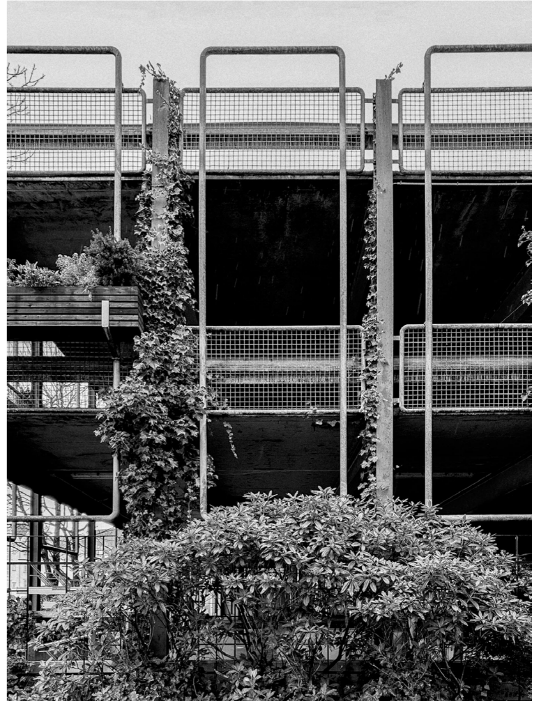
A green facade that contributes to creating a pleasant atmosphere.
