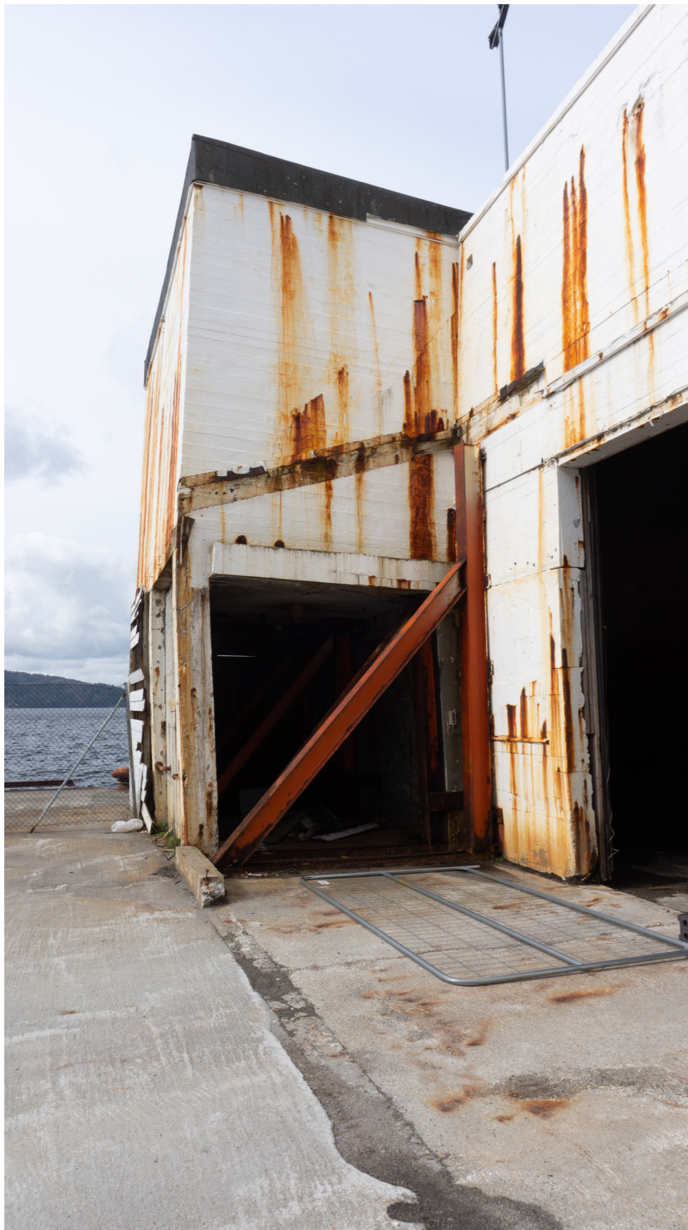
Weathered building, picture from site
